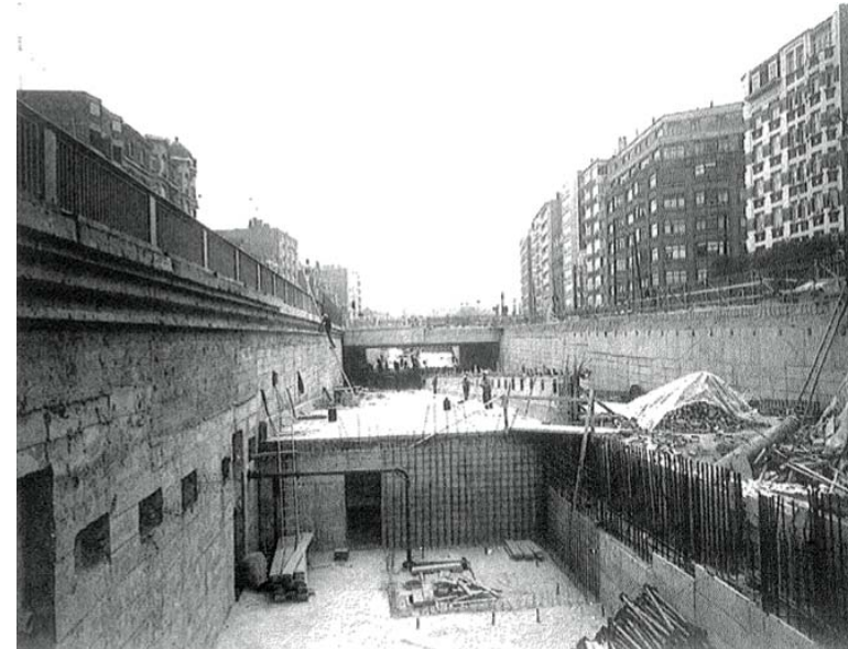
Figure 4 : Construction du tunnel Georges-Henri
